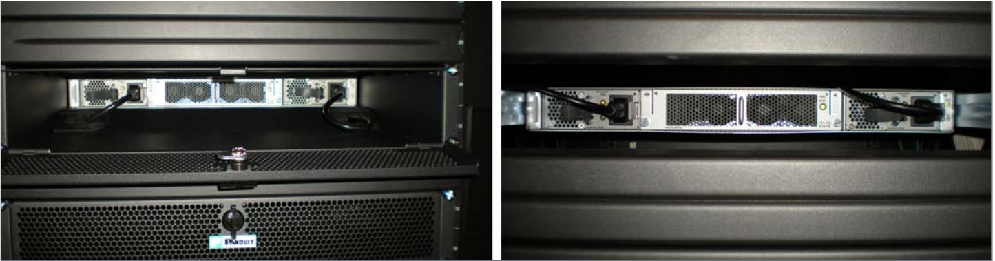
Figure 4.9. Server cowlings force air to flow through, rather than around servers. Left: server with cowling installed. Right: server without cowling installed. Photo by Michael Sheppy, NREL/PIX 19936
