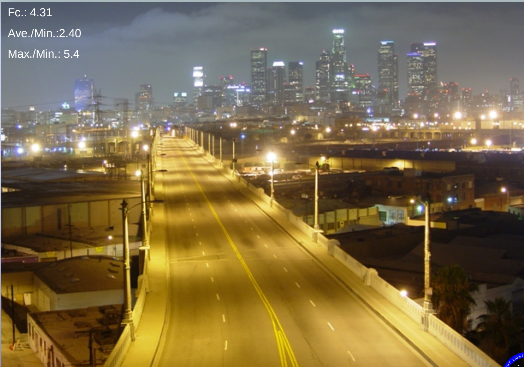
BEFORE – 200 W HPS (240 W) 6 th Street Bridge over Los Angeles River
