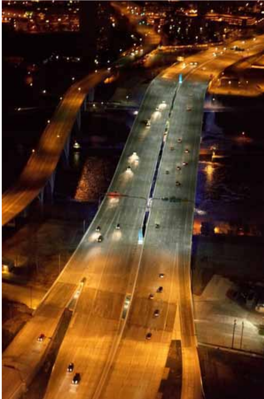
Figure 2.2. Aerial View of I-35W Bridge
