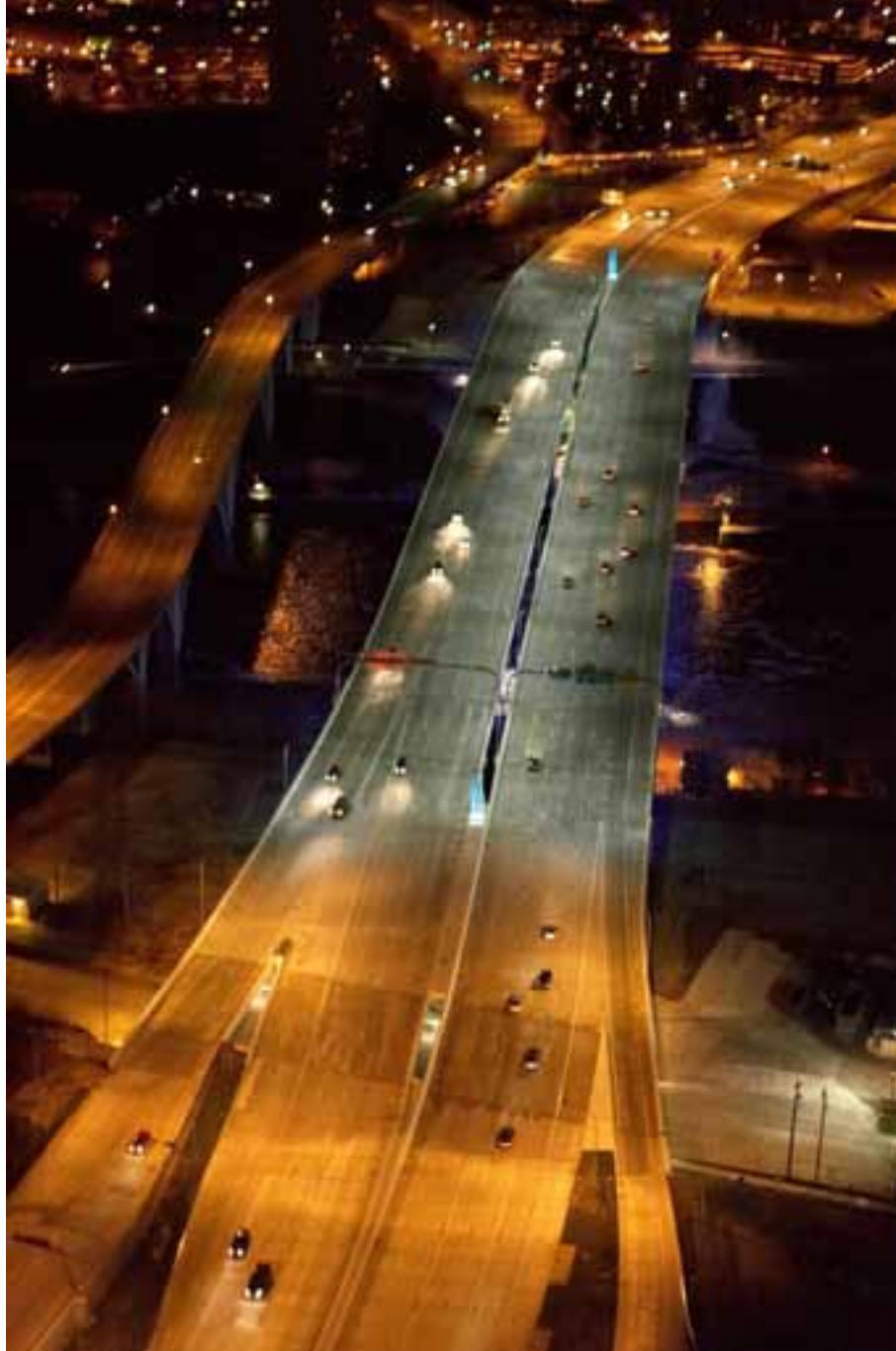
Figure 2.2. Aerial View of I-35W Bridge
