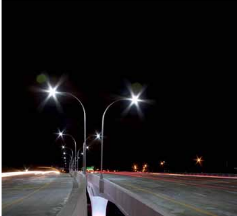
Figure 2.1. Luminaires installed on the I-35W Bridge.
