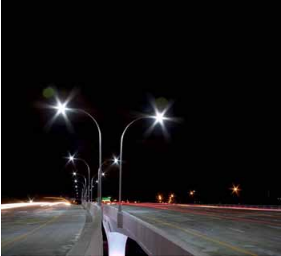
Figure 2.1. Luminaires installed on the I-35W Bridge.
