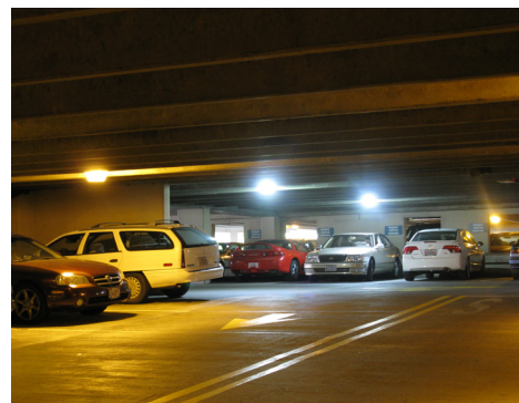
LEDs (middle two fixtures) replace high-pressure sodium lighting in this parking garage at the Providence Portland Medical Center. Photo courtesy of Pacific Northwest National Laboratory.
