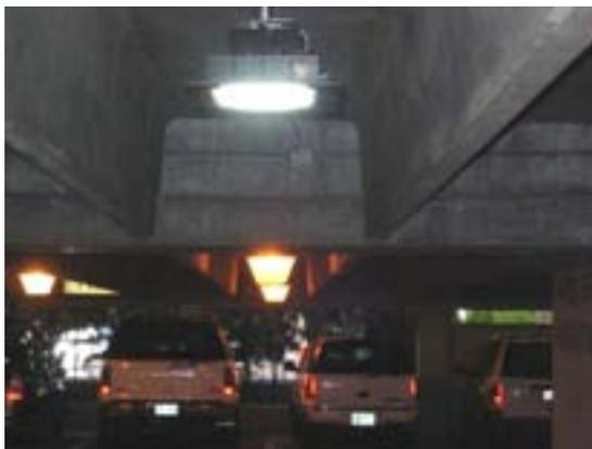
**Figure 3.5.** Installed LED Luminaire at PPMC Garage (Level B), with Security Camera in Background
