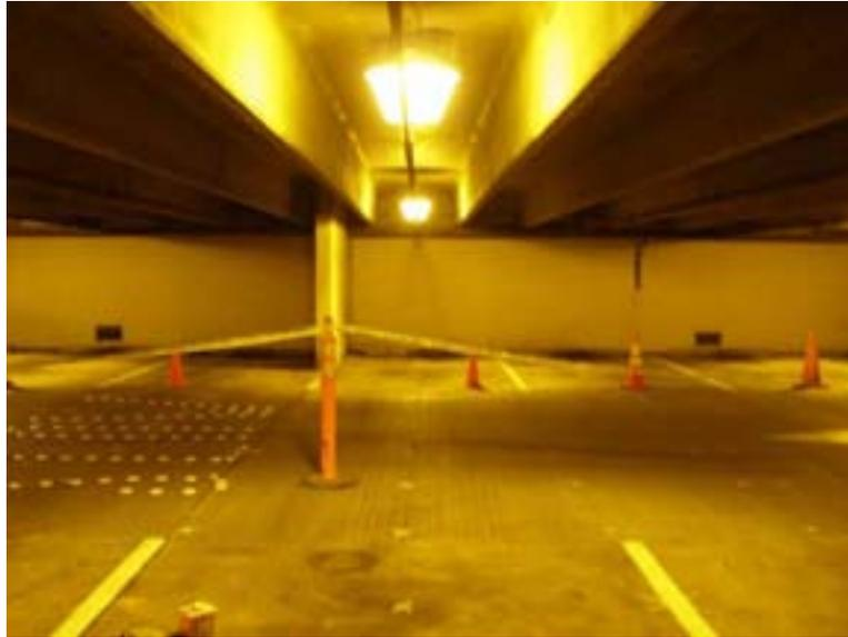
**Figure 2.5.** Crouse-Hinds HPS Luminaires at the PPMC Garage.
