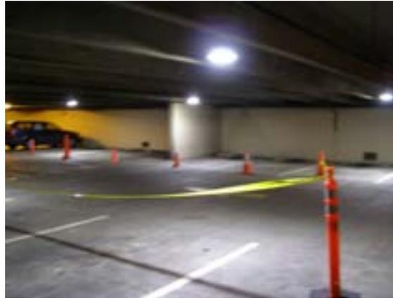
**Figure 3.3.** Installed LSG Low Bay LED Luminaires on PPMC Parking Garage Level A
