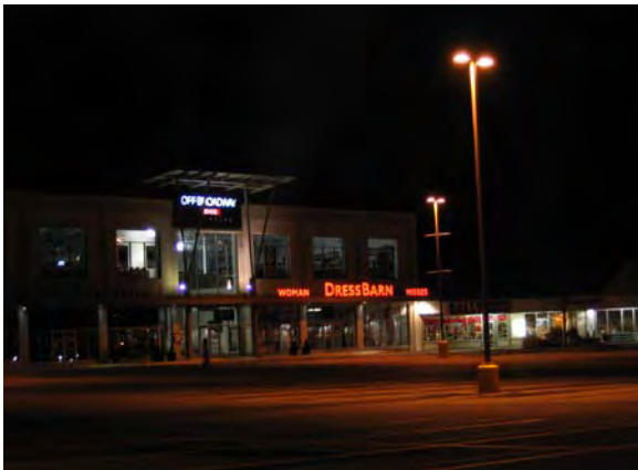
Figure 2.2. Original HPS Luminaires
