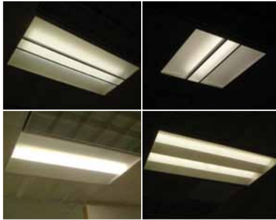
The four luminaires that were most-favorably rated for reflected glare all had diffuse lenses and seemed to have fairly uniform gradients across the troffer aperture.
