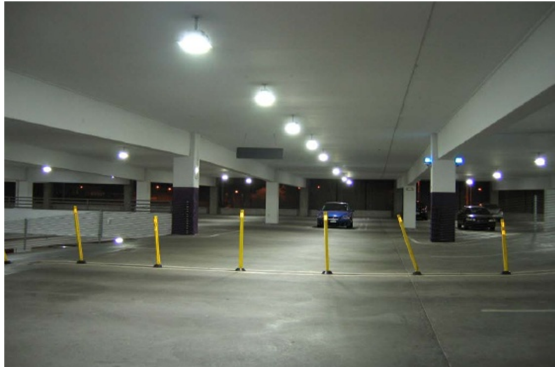
Arizona State University Parking Structure Courtesy of PNNL
