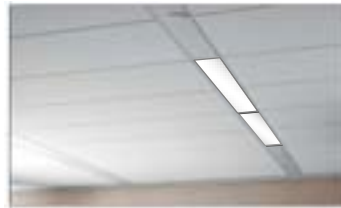
PHOLED Ceiling Lighting
