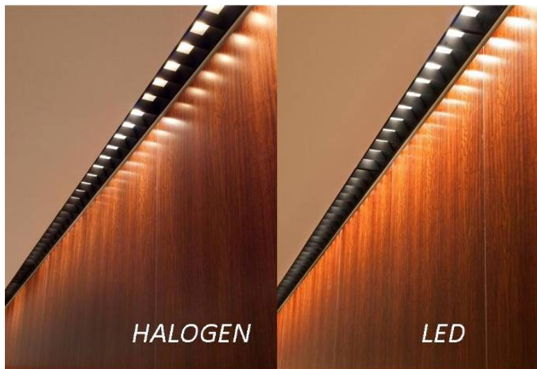
A comparison of LED and halogen products for the same application at the InterContinental San Francisco hotel
