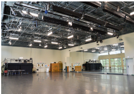
The Dance Studio, after the general lighting was replaced with 20 edge-lit LED luminaires. Photo by Stan Kaye.
