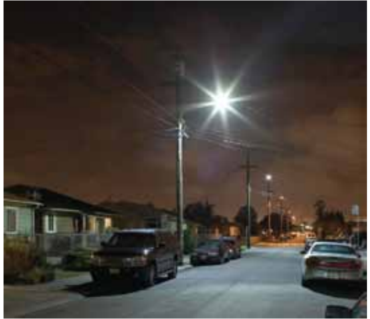
Demonstration in Oakland, California, with Beta LED streetlights (foreground) and HPS streetlights (background) Photo: Beta LED
