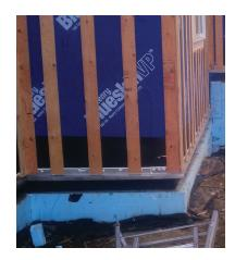
The exterior sheathing of the home was wrapped with a self-adhering vapor-permeable house wrap that serves as a weather-resistant air and water barrier. Furring strips were installed over this barrier allowing it to serve as a drainage plane for any bulk water that manages to get past the fiber cement siding.
