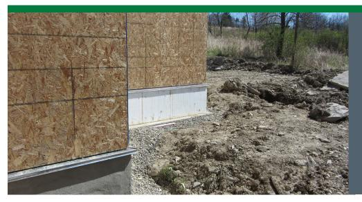
A shallow, frost-protected foundation saves excavation time and costs while insulating the homes' concrete slab foundations.
