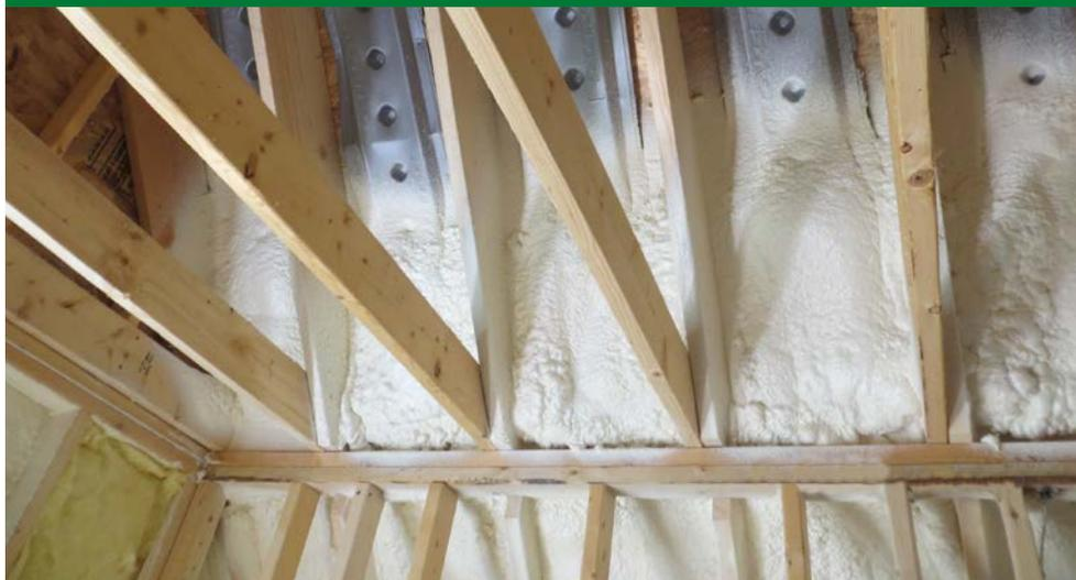
Closed-cell spray foam was applied to the walls up to and over the top plate in a “flash and batt” approach that used 1.5 inches of spray foam to air seal and insulate the wall cavities, which were then completely filled with 2 inches of unfaced fiberglass batt. An additional R-6.5 of foil-faced polyisocyanurate was installed as a continuous rigid foam sheathing on the exterior to reduce thermal bridging and provide a combined wall insulation value of R-25.
