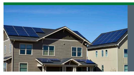
All of the homes in New Town Builders' communities at the Stapleton development in Denver feature solar panels along with the energy-saving features specified in DOE's Zero Energy Ready Home program. The 8-kW PV system provides more than enough power to meet the annual energy needs of this energy-efficient home, making this a true net zero energy home.
