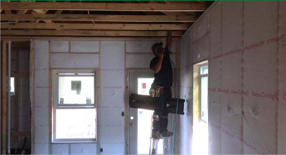
Palo Duro Homes achieves HERS ratings of 48 to 58 by stuffing walls with R-22 of blown fiberglass and carefully air sealing at top and bottom plates, around windows and doors, and at any outlets, wiring or plumbing holes.
