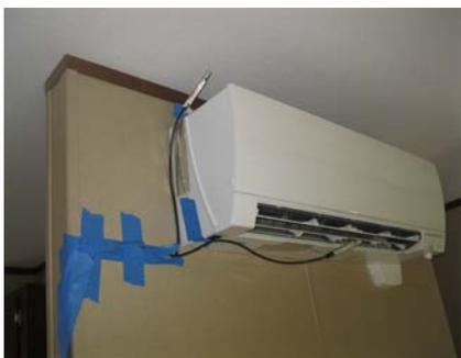
This single small mini-split heat pump (shown here in the prototype home with monitoring equipment attached) provides all of the heating and cooling the home needs with exceptional efficiency. No ducts mean fewer holes through the home's floor. Small thermostat-controlled fans inserted in the bedroom walls draw cool or warm air into those rooms when needed.
