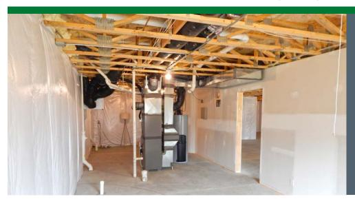
The high-efficiency furnace and heat pump water heater are located in a mechanical room in the insulated, unfinished basement.
