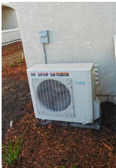
The air-to-water heat pumps provide efficient, combustion-free heating, cooling, and hot water.
