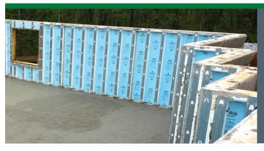
The home's basement walls are constructed of pre-cast concrete panels. The moisture-resistant walls have a continuous thermal barrier consisting of integrated rigid foam that covers the inside surface of the concrete panels and wraps around the concrete studs, behind the metal nailer facing, to stop heat transfer through the walls.
