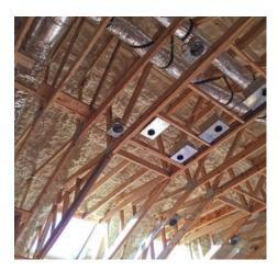
All ductwork is well sealed, insulated to an insulation value of R-8, and located inside conditioned space in the spray foam-insulated attic.
