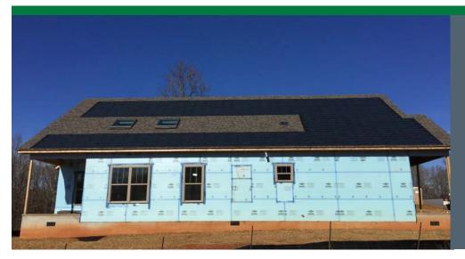
Solar electric shingles on the south-facing roof make this home a true zero energy home, generating enough electricity to meet the home's electricity needs over the course of a year. Whenever the solar power system provides more energy than the home needs, the home owners receive a credit on their electric bill for the excess power produced.
