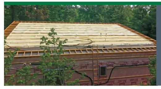
The home was insulated above the roof deck. After installing ice-and-water shield over the entire decking, the builder installed 1x4 purlins, which were set off from the decking using 6-inch sections of PVC pipe that were set upright. The purlins were screwed to the decking using very long screws that extended through the PVC sleeves. This provided space to install 5.5 inches (R-38.5) of closed-cell soy spray foam over the roof decking under the standing seam metal roof.
