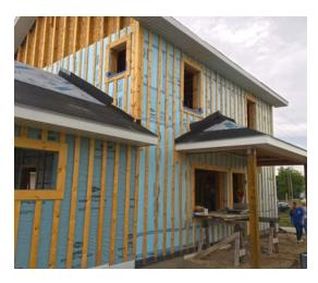
The 2x6 framed walls were filled with blown fiberglass and wrapped with R-20 of rigid foam. Furring strips provide an air gap under the fiber cement siding.
