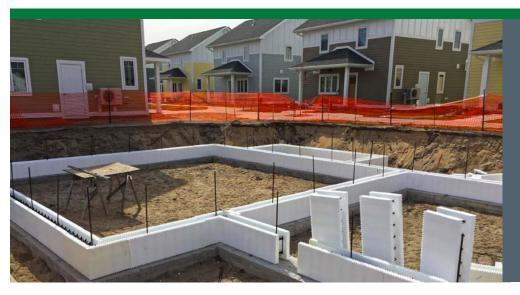
After excavating 60 inches, the builder poured concrete footings and constructed 54-inch-high insulated concrete form (ICF) footing walls, then backfilled the space within the walls with dirt to within 12 inches of the top of the ICF walls. The packed dirt was covered with three 2-inch layers of rigid EPS foam board, providing R-30 of insulation under the 4-inch concrete slab while the ICFs provide R-20 of slab-edge insulation.
