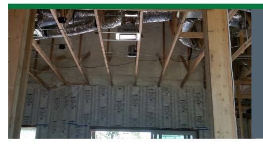
For efficient and comfortable heating and cooling, all of the home's ductwork is located in the conditioned attic. The attic is insulated to an insulation value of R-38 with open-cell foam. The home's walls are insulated using a radiant barrier insulation that blocks heat from the sun and keeps it from entering the home.
