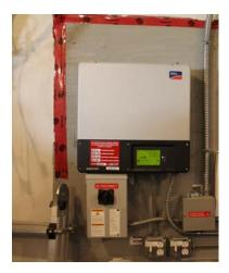
The photovoltaic system includes two inverters that are tied to the grid but also wired to provide electricity to one outlet each should the grid go down.
