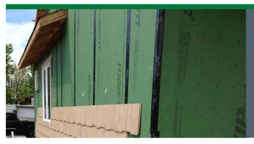
The insulated sheathing is taped at the seams to provide a continuous air barrier, thermal barrier, and drainage plane behind the siding. No house wrap is needed.
