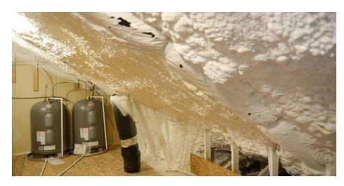
Spray foam covers the attic ceiling providing an insulated location for the HVAC ducts.
