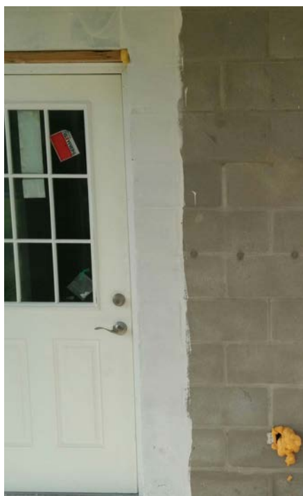
A paint-on waterproofing compound provides seamless protection around doors and windows.
