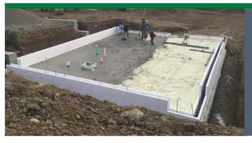
All of Greenhill's homes are constructed with insulated concrete forms (ICFs), which not only provide energy-efficiency advantages, but are also rated to withstand hurricane-force winds and earthquakes.
