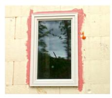
A thick waterproofing paste is applied around window and doors openings to provide a seamless layer of protection against rain intrusion. With the seams sealed, the ICFs provide a water-resistant barrier so no house wrap is needed.
