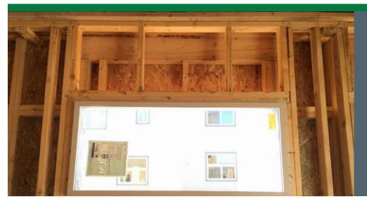
Thrive's Courtyard townhomes start with double-wall construction which provides 9.5 inches of space for blown fiberglass insulation. Advanced framing techniques like open headers, two-stud corners, and ladder blocking at wall intersections allow even more space for insulation. ENERGY STAR-labeled windows provide daylighting while their low-emissivity coatings help prevent heat loss and unwanted solar heat gain.
