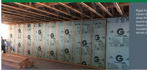
Rigid foam lines the basement walls and covers the exterior above-grade walls to wrap the house in a blanket of continuous, sound-proofing, heat-blocking insulation. Seams are taped in the above-grade insulation so that the rigid foam also serves as an air- and water-barrier.
