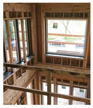
Dwell Development constructed the energy-efficient home with 12-inch-thick double-stud walls that were air sealed on the exterior and at all window openings with a dark roller-applied liquid flashing. The walls will be packed with R-44 of dense-packed cellulose.
