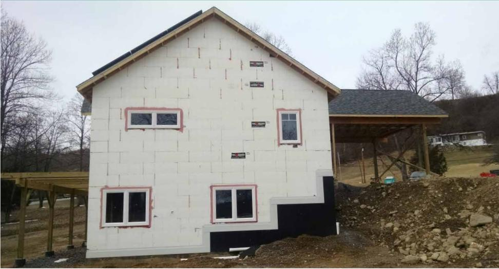
Like a Styrofoam cooler, this Greenhill Contracting home is wrapped in foam insulation, with 4.5 inches of closed-cell spray foam under the slab and 11.25-inch-thick R-22 ICF block walls. The underside of the roof deck is covered with 10.5 inches of open-cell spray foam plus 2.5 inches of closed-cell spray foam to provide an R-65 insulated attic.
