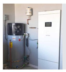
An efficient heat pump water heater provides hot water for the all-electric home while the 10kW battery storage system covers late afternoon energy demands.
