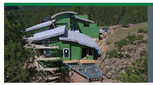
A self-adhered membrane completely covers the roof decks and fascia to help prevent water leakage under the metal roofs. The coated wall sheathing will be covered by two inches of rigid foam.
