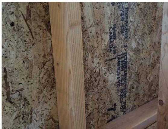
The exterior wall is a double wall consisting of two 2x4 24-inch on-center advanced-framed walls with a 2.5-inch gap between creating a 9.5-inch cavity that was dense packed with blown fiberglass to provide a continuous R-41 layer of thermal protection around the home.
