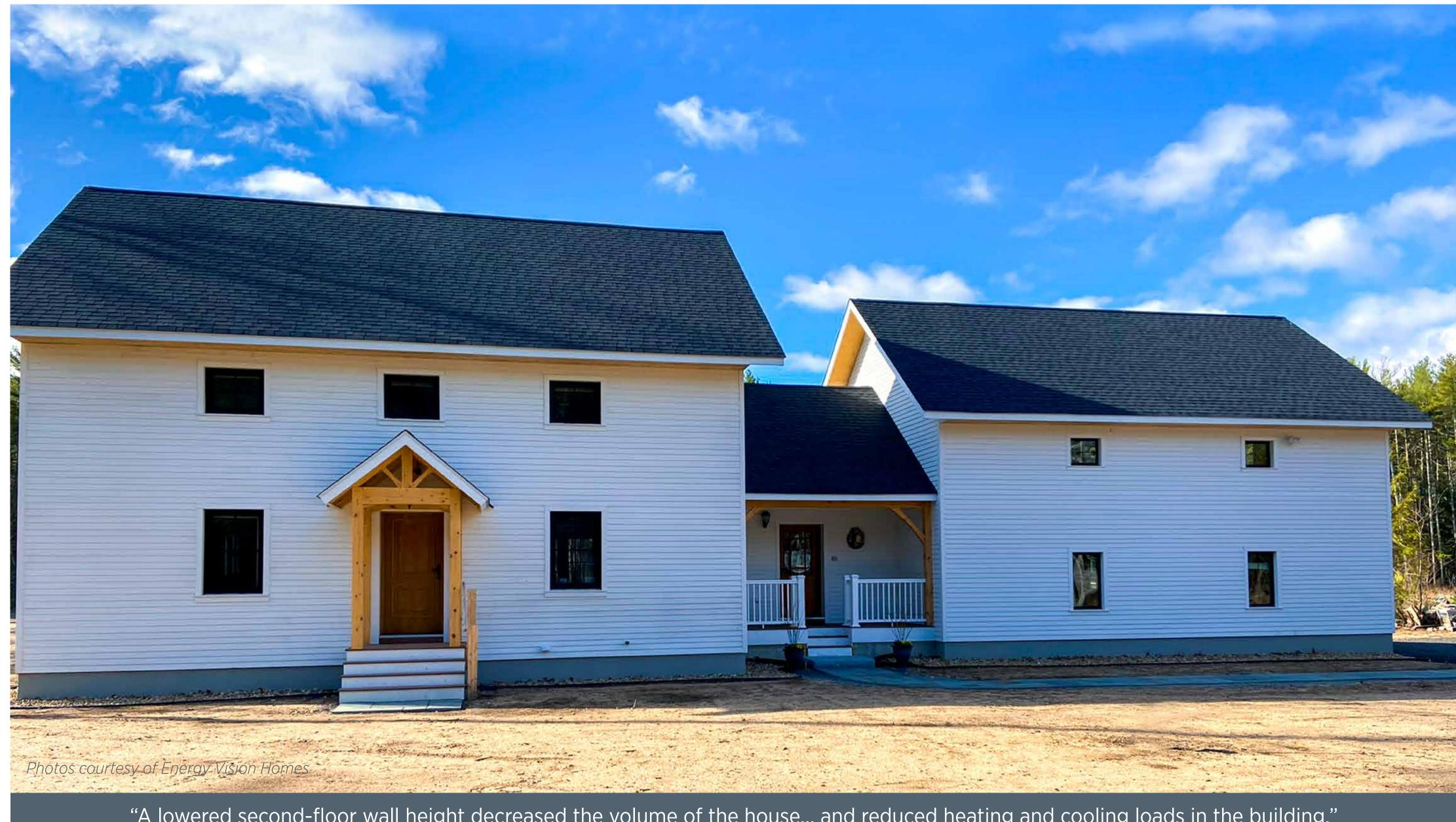
"A lowered second-floor wall height decreased the volume of the house... and reduced heating and cooling loads in the building."
