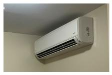
The home's air-source ductless mini-split heat pump has one outdoor variable-speed compressor and two indoor air handlers and provides very efficient heating and cooling (14 HSPF, 33 SEER).
