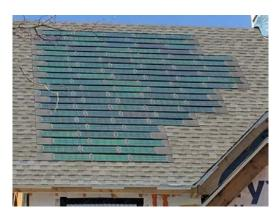
Murphy Brothers installed a 4.5-kW photovoltaic system using PV shingles that integrate into the roof for a lower profile than raised panels.
