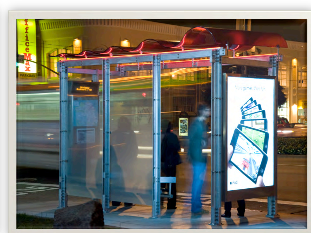
San Francisco Municipal Transportation Agency Bus Shelters by Lundberg Design using Konarka Power Plastics. Plastic photovoltaic roof produces enough power to keep the shelter, with a wi-fi router, LED bus schedule updates, lighting, and advertising, day and night. Pictures from ( http://greenarchitecturenotes.com/2010/01/san-francisco-municipal-transportation-agency-bus-shelters-a-new-design-technology-business-model-for-green-architecture/ ).
