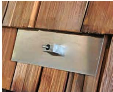
Figure 6. Penetrating mounts
