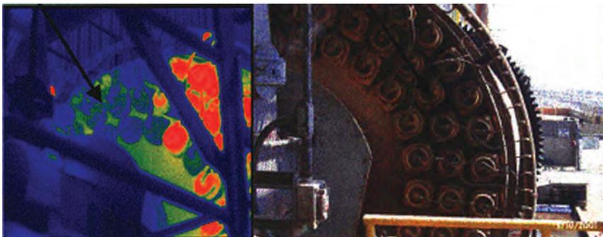
**Figure 6.2.9.** Inoperable steam heaters seen by cooler blue areas when compared to the operating heaters warmer red or orange colors.
