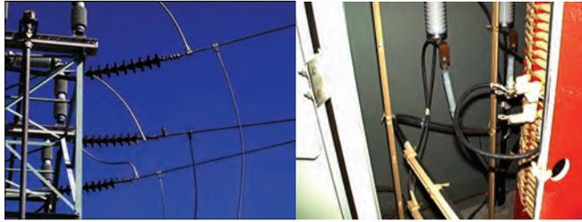
Mechanical devices are not the only sources of ultrasonic emission. Electrical equipment will also generate ultrasonic waves if arcing/tracking or corona are present.
