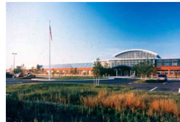
A study of the new headquarters for the Herman Miller furniture company indicates that the new sustainable building had positive impacts on occupants' well-being, job satisfaction, feelings of belonging, and other aspects of work life that affect individual job performance. Productivity measured by the company's own total quality metrics increased when employees moved into the new space,
