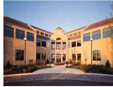
When workers at the West Bend Mutual Insurance Company moved into their new building with personal controls for their workstations and other sustainable features, productivity increased 16%.
