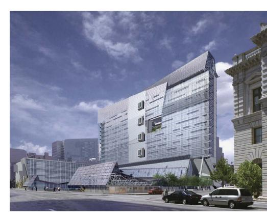
Automated operable windows and night vent cooling -> no mechanical cooling for perimeter offices
