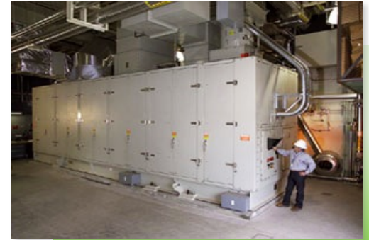
4.4MW Solar Mercury 50 Turbine Generator
