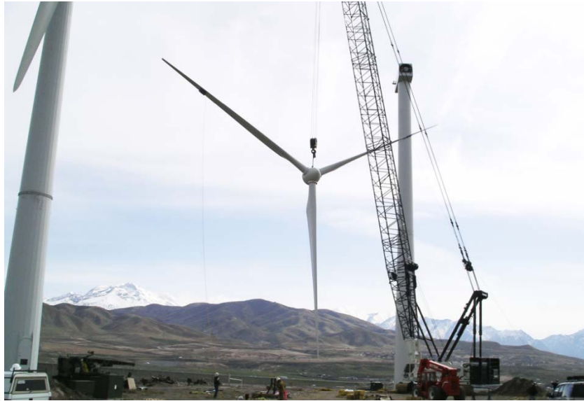
Figure Vestas V-47 installation at Camp Williams in May 2005
