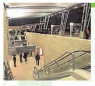
The Pentagon metro entrance facility's canopy skylight is constructed of self-bleaching, Teflon coated, fiberglass fabric and offers three-sided weather protection.
