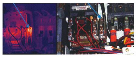
Figure 6.2.5. Overloaded contacts show different temperature profiles indicating one contact seeing much greater load, a potentially unsafe situation.
