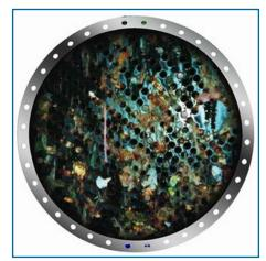
Figure 10. Biofouled Heat Exchanger (Source: Taprogge GmbH).
