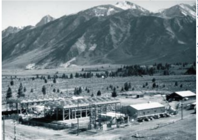
Geothermal Resources Council/PIX00062
